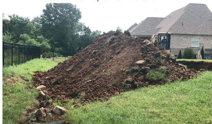
The dirt removed from the hole will be placed in close proximity to the pool so that it will be easier to move by the homeowner once the pool project has been completed.
