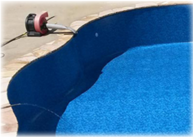
Wrinkles in liner during filling process are common
