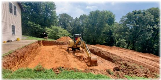
**Pool Walls:** Inground vinyl lined pools will be set with bracing attachments and will have a concrete footer poured. If concrete has to be pumped for the footer or walls there will be an additional charge.
