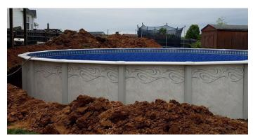
This pool had a very small slope, but you can see how much dirt is left behind. Additional excavation, grading and dirt work beyond that which is required for leveling the pool site is available by bid only and made prior to install date.
