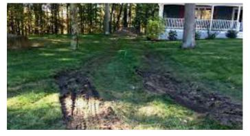
It is very common with the heavy equipment used to dig your pool coupled with wet or softer yard conditions that ruts can form around your property. Our builders will try and use the best route to eliminate this, however most times there will be some work on the homeowner to repair or fill the ruts. The excess sand and dirt from your pool build should provide the material needed in the damaged area.
